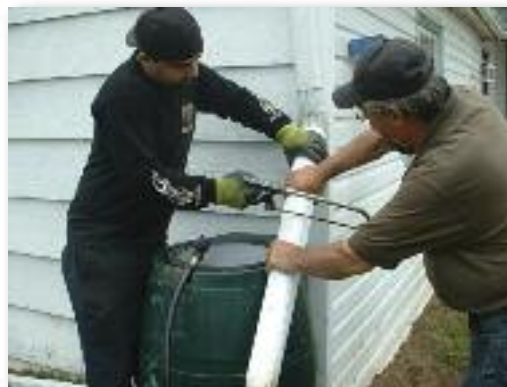
Rain Barrel being installed
