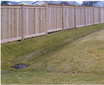
Typical backyard swale with a drain.
