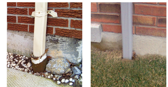
If your downspout looks similar to these, chances are it is connected to your weeping tile or the municipal sanitary sewer system and should be changed.
