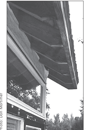
Open eaves, vents not screened (6 pts)
