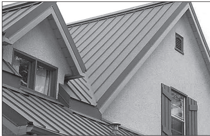
Metal, clay tile, asphalt shingles, or non-combustible material (0 pts) – the most fire resistant and remain effective under severe fire exposure.
