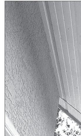
Closed eaves, vents screened with 3-millimetre mesh and accessible (0 pts)
