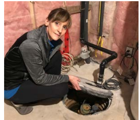
Councilor Coburn testing the sump pump
