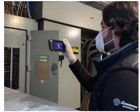
A Wawanesa Loss Control Representative conducts an Infrared Thermography scan on an electrical panel during a commercial inspection
